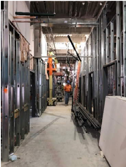
Looking down the long corridors of the upper level Clinic / Med Surge addition. Many lifts are being utilized to installing the drywall topping out in these corridors. In the next weeks the full drywall installation will begin and MEP above ceiling rough ins.
