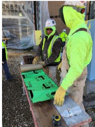
The next step is measuring out and installing the waterproof membrane (the green adhesive paper pictured above) and apply a sealant to the densglass.
